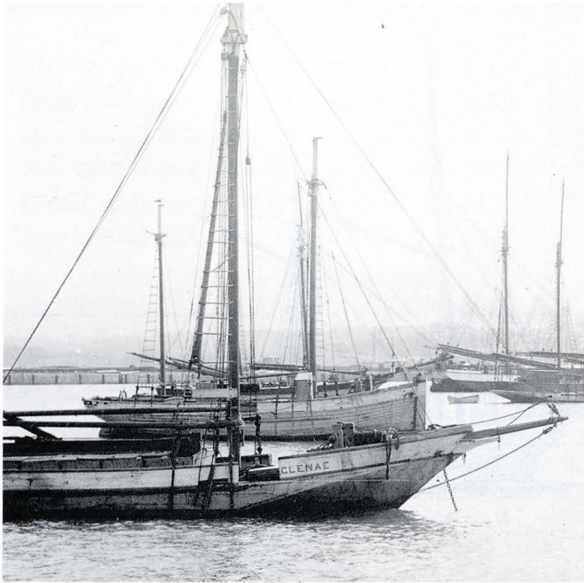
The GLENAE, a small hold ketch — note the hatches each side of the centrecase (D. Darroch, Omaha, 1904; 57.7 x 16.4 x 3.1 ft). (A.N. Breckon, C.W. Hawkins Collection)
