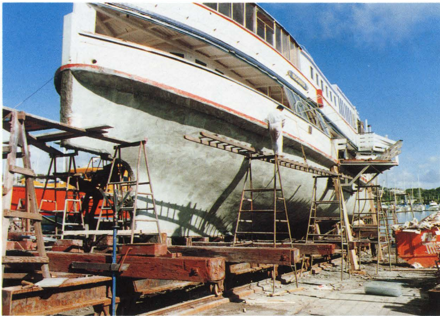
The completed ferrocement skin, awaiting epoxy paint.
