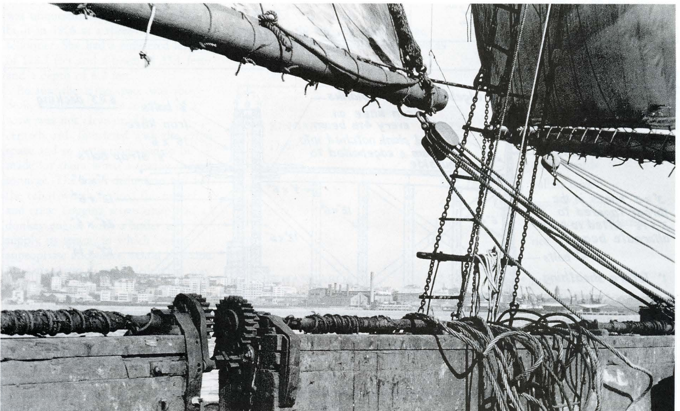
The twin centreboard cases of the RANGI, showing the geared winding shafts for hoisting, with pawl and ratchet.
