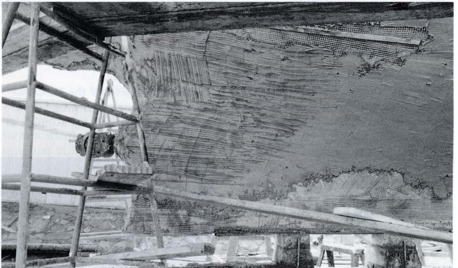
Galvanised mesh in place and ready for plastering.
